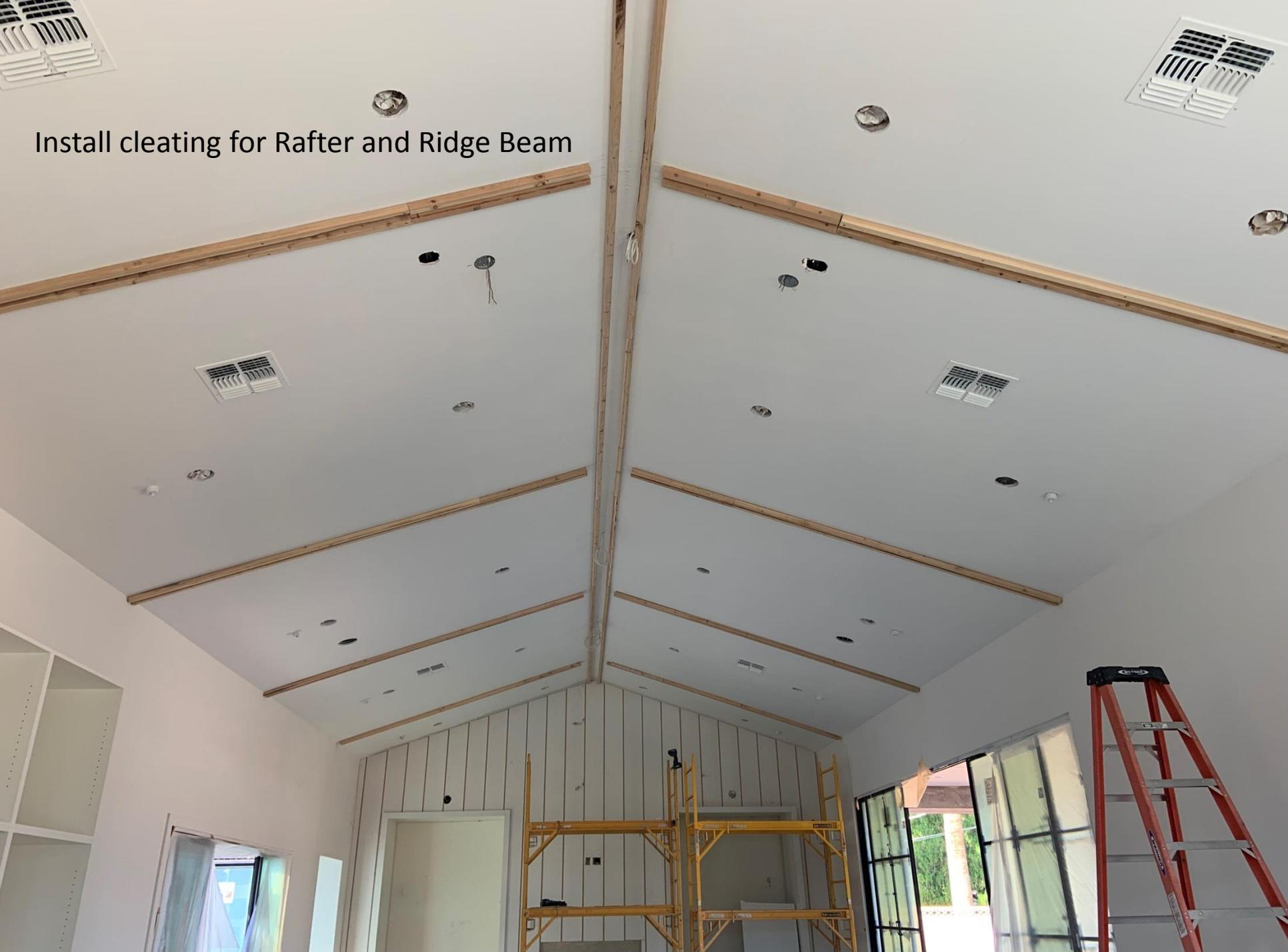
Install cabling to structural blocking in ceiling. Cut holes in bottom of Ridge Beam and install ridge beam.
