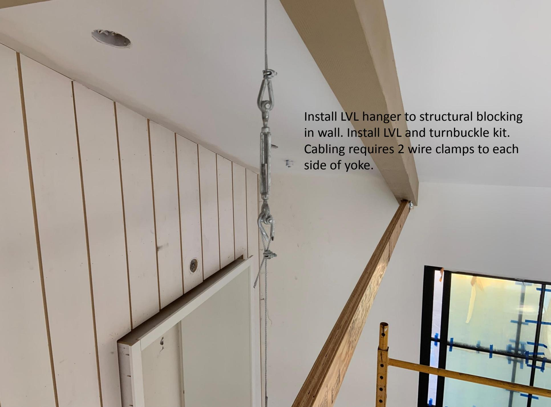
Install LVL hanger to structural blocking in wall. Install LVL and turnbuckle kit. Cabling requires 2 wire clamps to each side of yoke.
